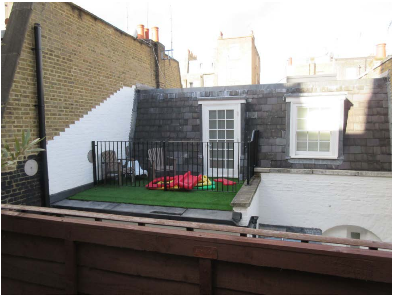
View of existing terrace from rear of 14 Chester Street
